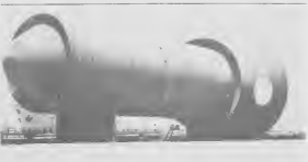
NO, NOT a missile bound for Cape Kennedy, but a new internal section for the PCAR reactor. The 158,000-pound section will be installed during the shutdown scheduled for October. NO, ENKARI no ta un cohete cu destino pa Cabo Kennedy, pero un seccion interno pa e reactor di PCAR. E seccion di 158,000 libras lo ser instalá durante e periodo cu e planta lo baha na October.
